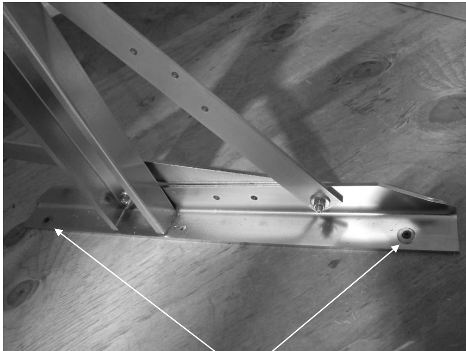
Attach steel foot to floor at front and back holes using concrete screws and ¼" flat washers. Figure 8.
